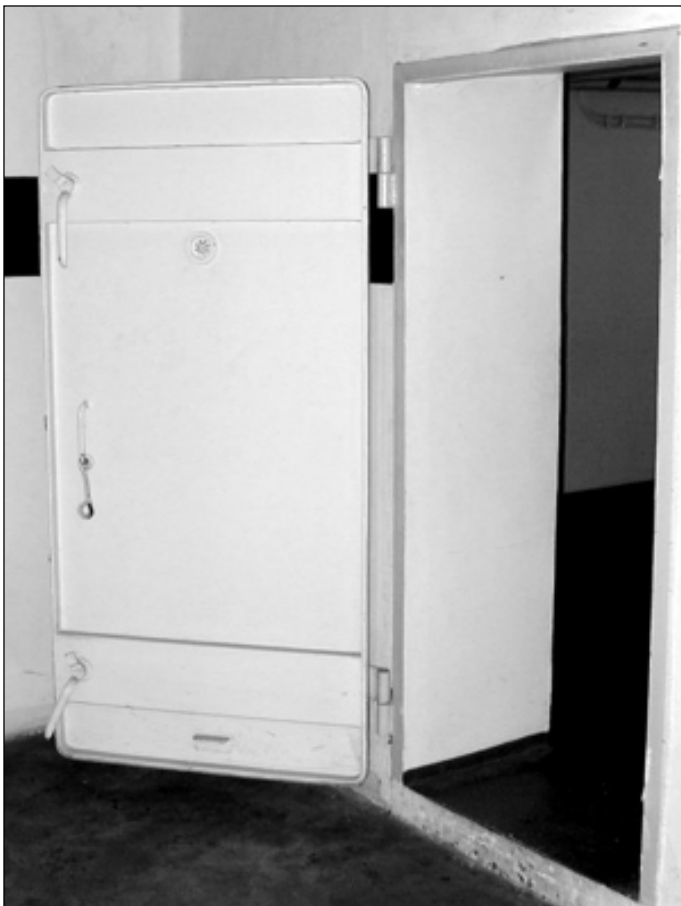
Standard gas tight air raid shelter door; peephole with grill
