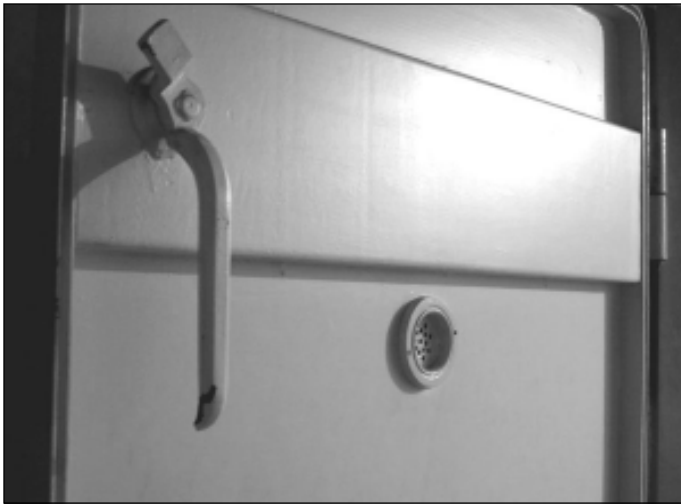
Standard gas tight air raid shelter door; peephole with grill
